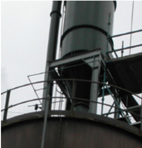
Silo Filter remotely monitored by a networked Electrodynamic System
