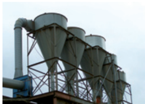
De-barking and chipper cyclones monitored by insulated Electrodynamic sensors
