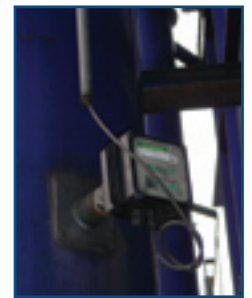
Electrodynamic Sensor installed in bag house outlet
