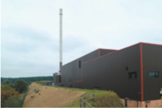
Biomass power plant monitored by an Electrodynamic Sensor and Filter Management System
