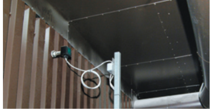
Electrodynamic sensor mounted in chamber wall
