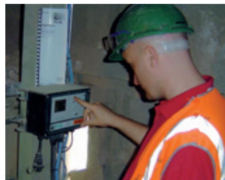
PCME instruments offer easy set-up/ interrogation of monitors either locally or remotely by either modubs /4-20mA outputs or via Ethernet, GSM & Web connectivity
