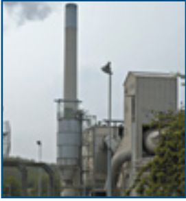
A Cement Kiln Baghouse incorporating an Electrodynamic filter management system
